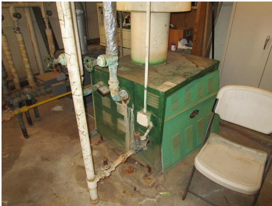
View of green boiler with white asbestos containing insulations inside. This material is assumed to contain asbestos based on previous sample results. No Samples were collected during this inspection.
