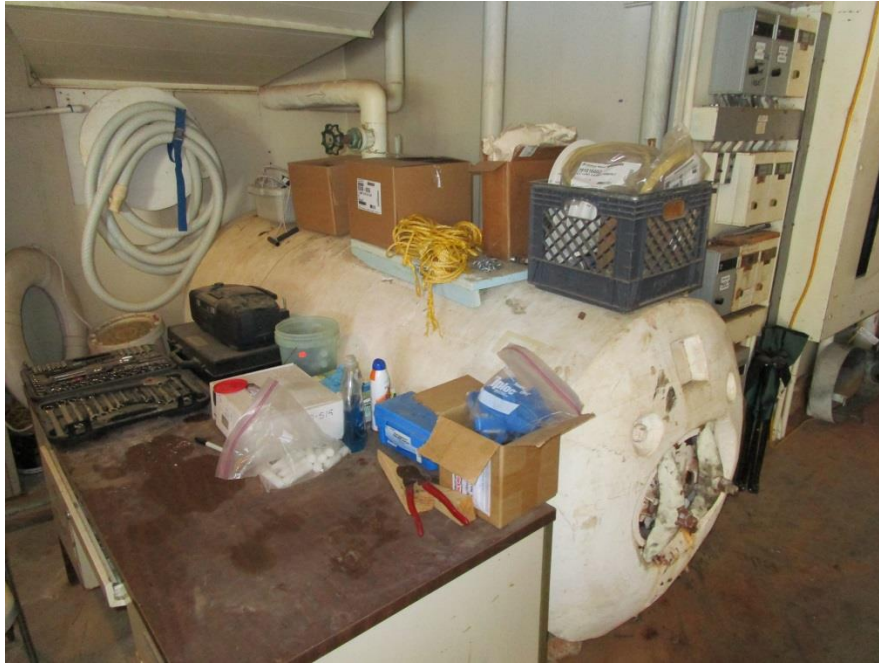
View of non-asbestos containing boiler insulation. Two bulk samples were collected as part of this assessment and two samples were collected as part of a previous assessment.
